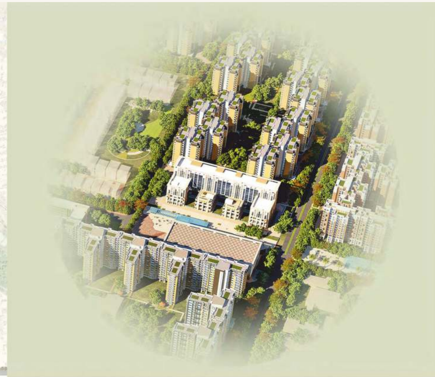
Direct Connectivity from Sarojini Nagar Metro Station
